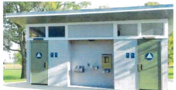
Public Restroom, El Sereno Park, California
